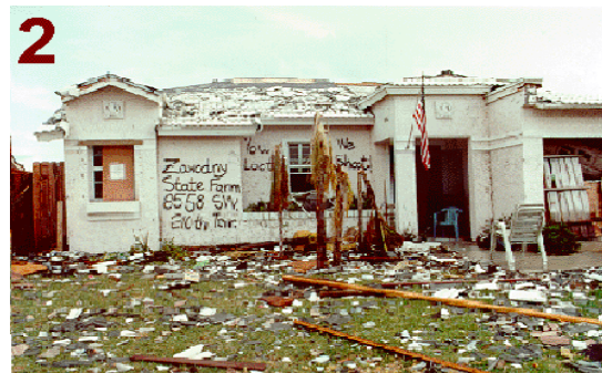
MAJOR DAMAGE HABITABLE
