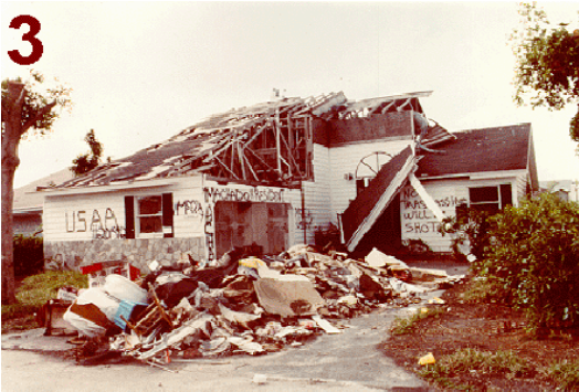
MAJOR DAMAGE UNINHABITABLE
